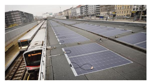
Our first pilot project was implemented in Vienna. As part of its environmental efforts, Wiener Linien launched a unique pilot project: The first-time installation of special photovoltaic films on the roof of the underground station in the Ottakring district. >> Read more <u>HERE</u>!
