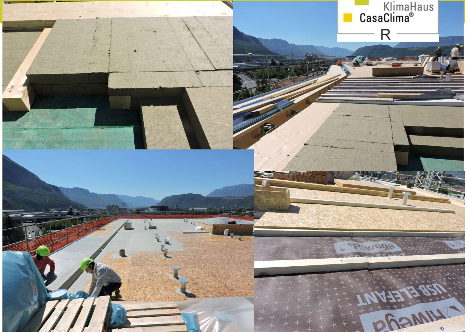
Roof insulation
