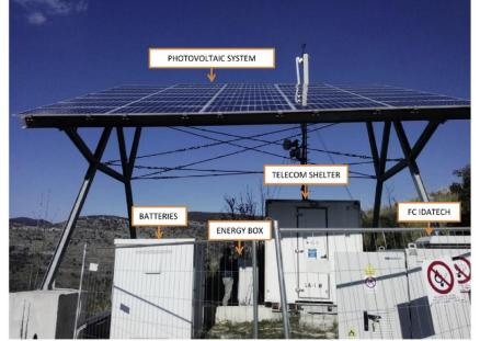
Installation of the FC system in Fiano Romano (site #2) from Cordiner, Mulone et al., Applied Energy, 192, 2017
