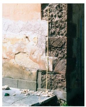
Images 3, 4: Patterns of acid rain on sandstone and of efflorescence both on rocks and on mortar
