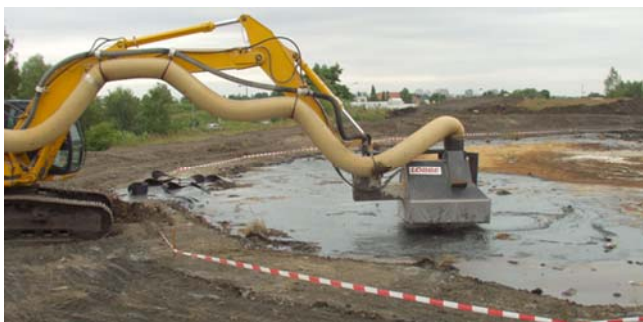
Fig. 16: Pasty tar was solidified with calcium carbonate and excavated
