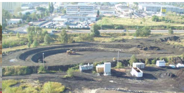
Fig. 17: Former tar ponds get filled up and covered
