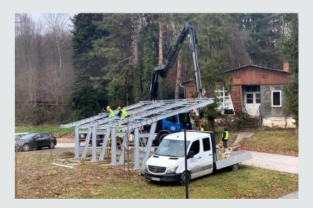
Figure 2: Canopy construction Source: REGEA 2021.
