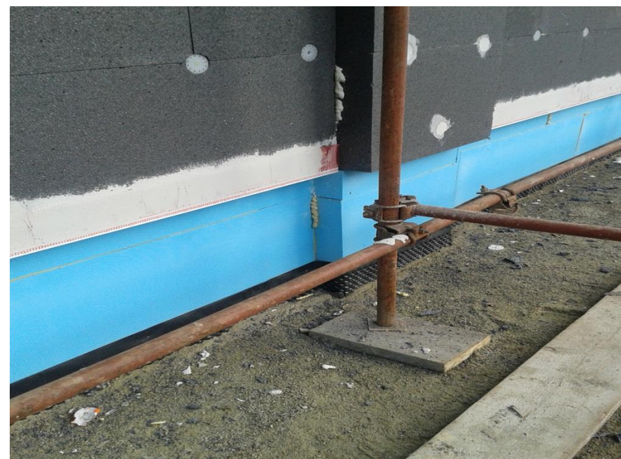
2. Thermal insulation of the walls above the foundation as a part of the ETICS system (boards of a extruded polystyrene) 10 cm;
