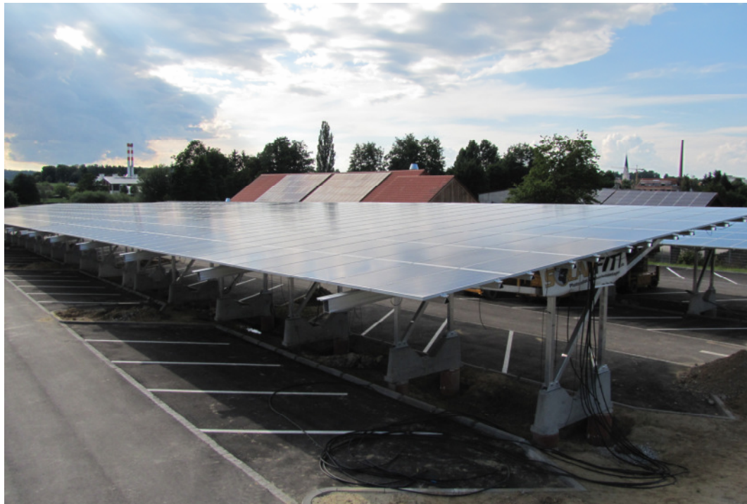
Photovoltaic plant: Solar car port, 284 kWp, => ~75 households in PAF
