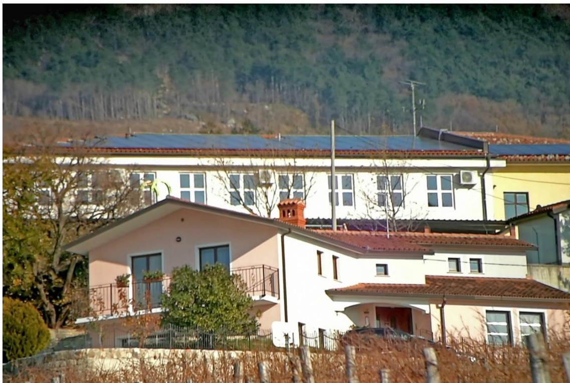
Image 32: Solar power plant in Budanje, Source: Luka Cerlevaris
