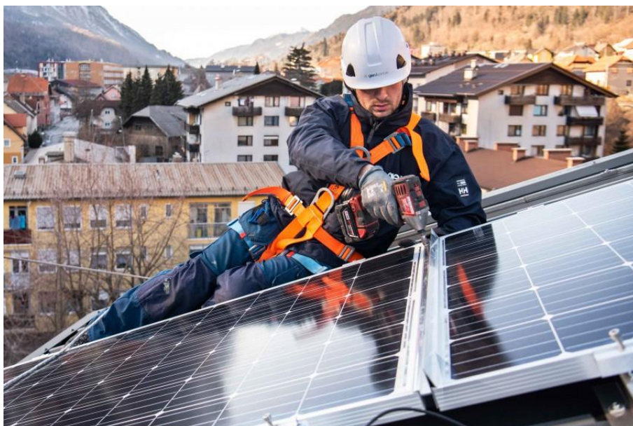
Image 31: Installation of solar panels, Source: GEN-I
