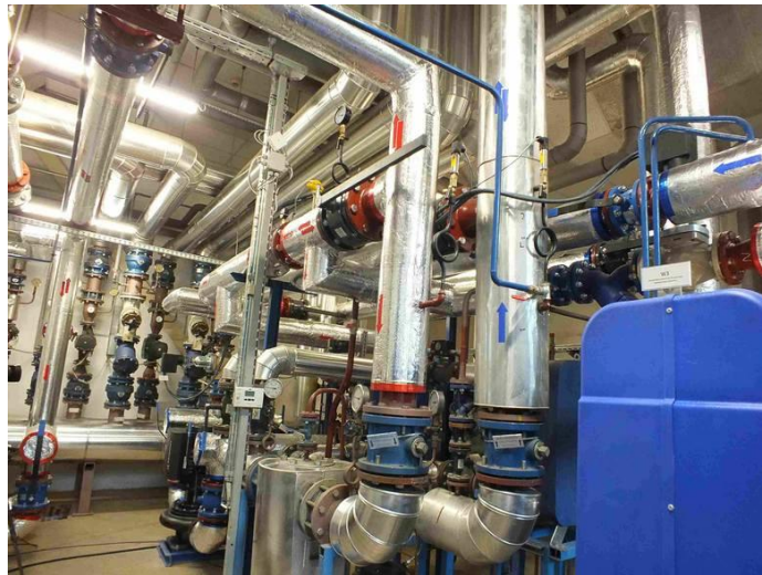
Image 23: Waste heat recovery installation, Source: Celsius Sp. z o.o., Kazimierz Cuch
