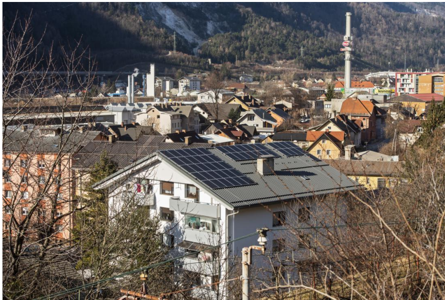
Image 30: The first solar power plant GEN-I Sonce on a multi-apartment building in Jesenice, Source: GEN-I
