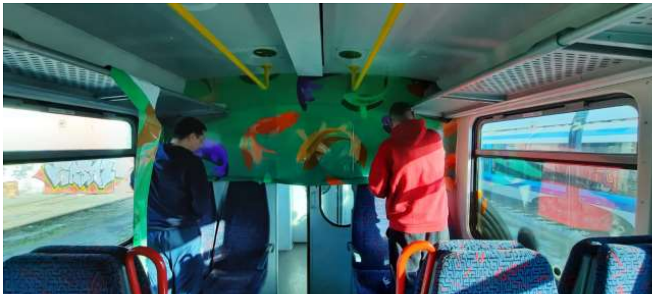
Fig. 11: Setting up self-adhesive foils in the train
