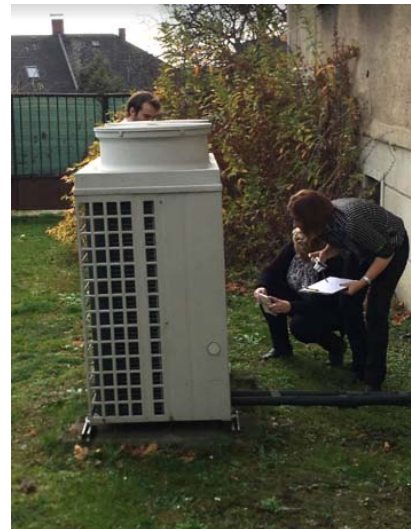
Figure 6 Inspection of a cooling station
