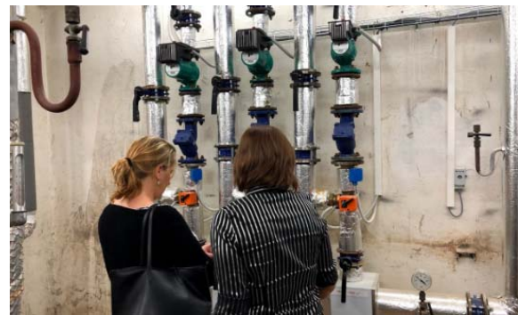
Figure 3 Inspection of a heat exchange substation
