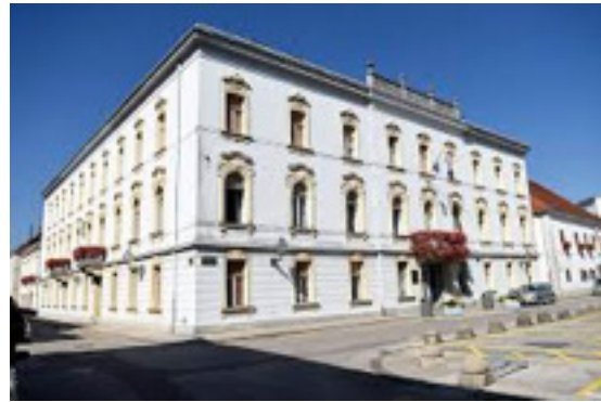
Pilot building - The City Hall building, Banjavciceva 9, City of Karlovac
