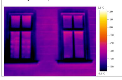
You can see that the temperature of the windows are almost the temperature of the outside air which means that windows are not causing any heat losses.
