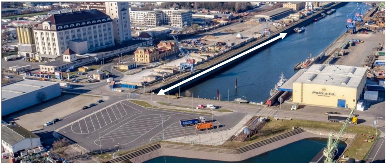
Figure 6: View of the south bank with marking of the track area intended for trailer handling; source: SBO
