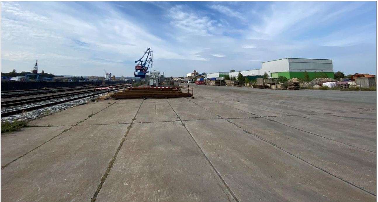
Figure 12: Transshipment area north bank (looking west)
