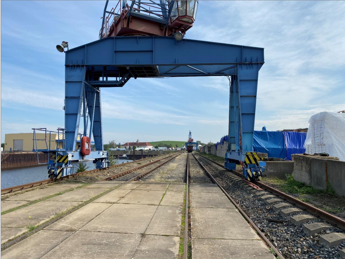
Figure 11: South bank, track area (facing east)
