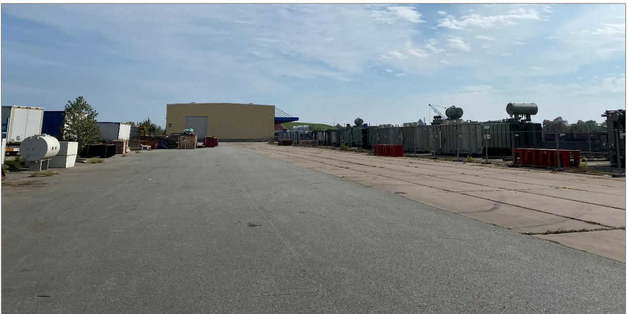
Figure 13: Transshipment area north bank (looking east)
