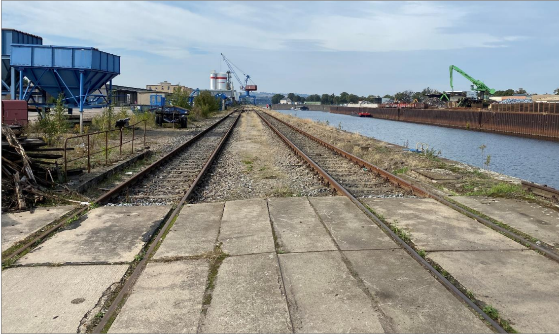
Figure 10: Track area (facing west)
