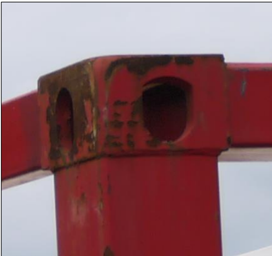
Figure 9: left side: upper corner castings, right side: twistlocks 2
