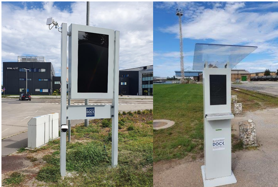
1. Figure Installed devices for the intelligent access and traffic management system
