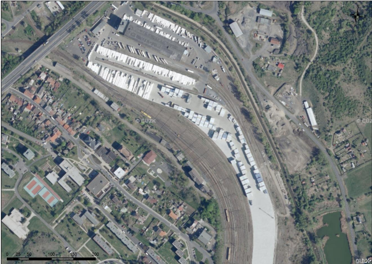
Picture 6: Intermodal terminal Obrnice
