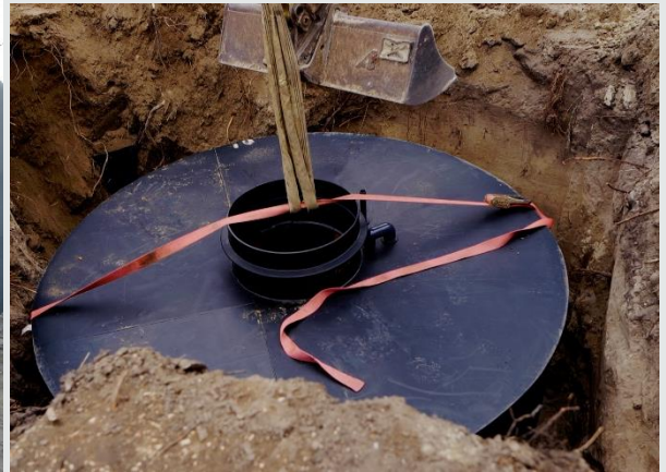
Water tank installation
