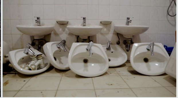
Indoor construction works
