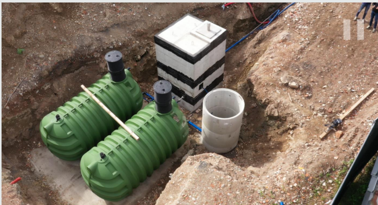
Figure 1: Underground storage tanks and equipment shaft during construction
