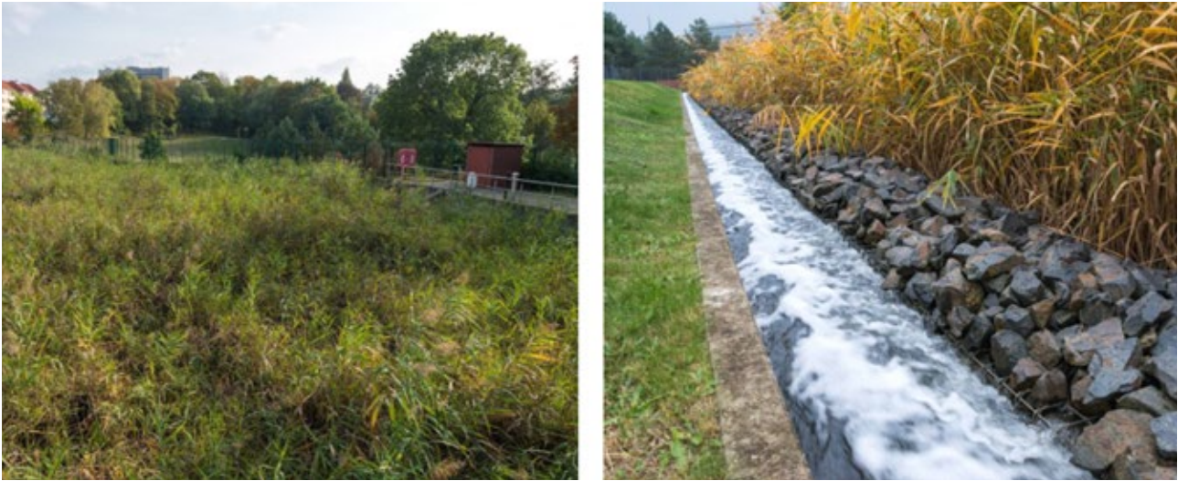
Figure 25: Retention soil filters in Berlin (Photo: Andreas Süß).
