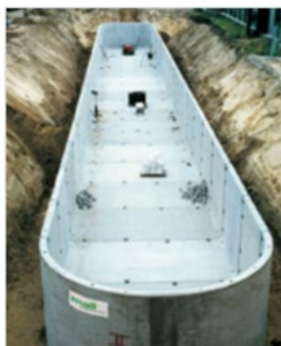
Reinforced concrete cistern (24 - 100 m 3 ) (Mall)
