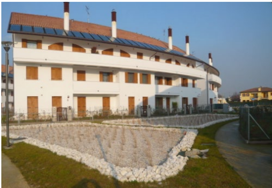
Figure 17: HF system for the separation, treatment and reuse of greywater for toilet flushing in a residential area in Preganziol (TV - Italy) 45 .
