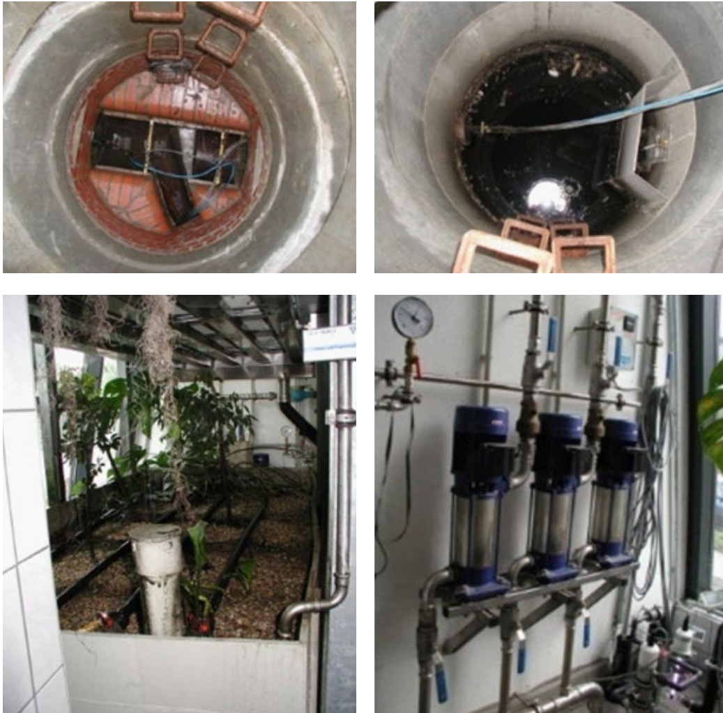
Figure 47: Rainwater sewer with switch diversion (above) and planted soil filter inside the building (below).
