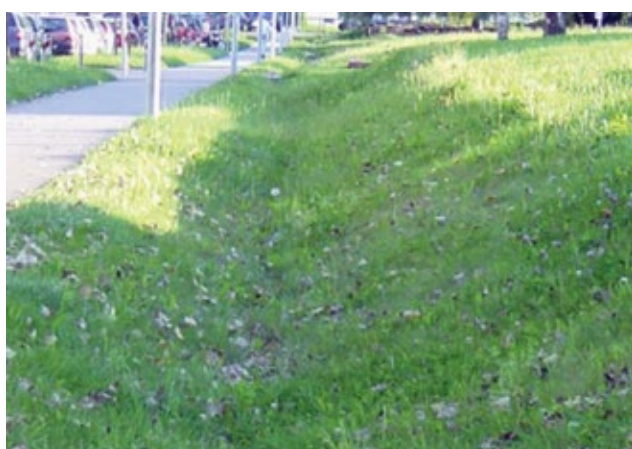
Figure 35: Vegetated swales (Büro Grimm).
