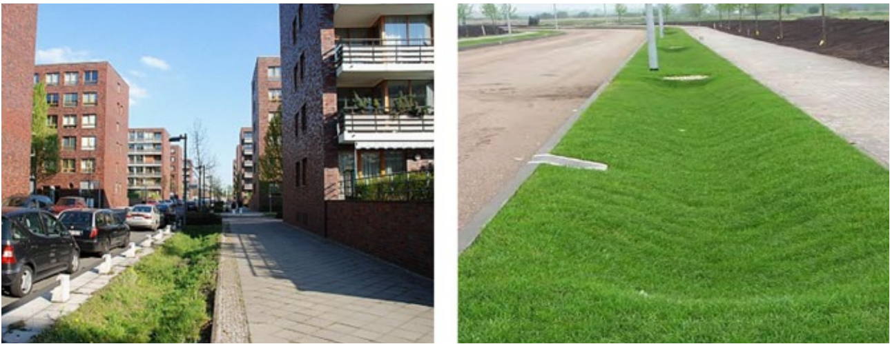
Figure 44: Swale-trench systems in Berlin (Sieker).
