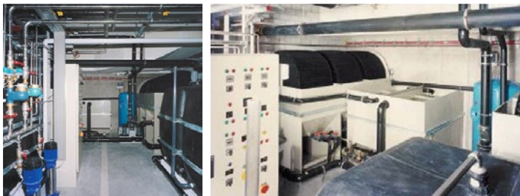
Figure 28: The greywater recycling system with the 6 RBC modules and the post-sedimentation tank.
