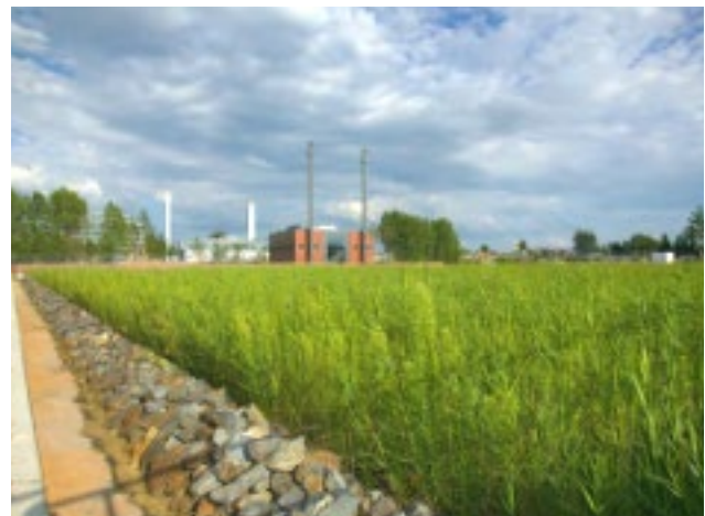
Figure 56: Retention soil filter (RSF) at Berlin-Adlershof (Source: BWB).
