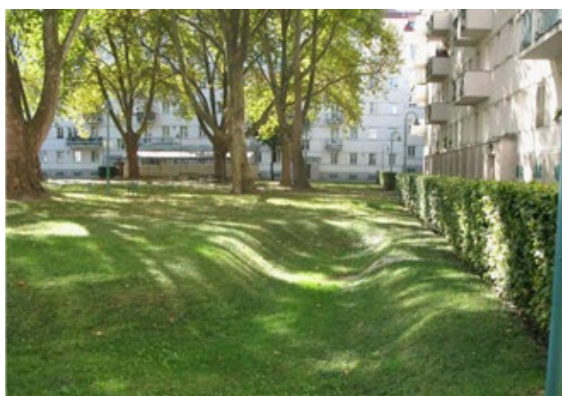
Figure 36: Swales in residential areas (Sieker).
