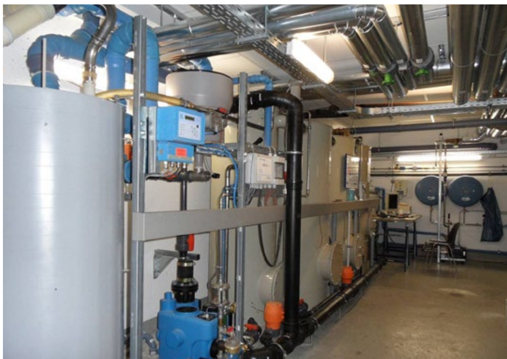
Figure 24: The greywater recycling system including heat recovery from greywater in the cellar of the building.
