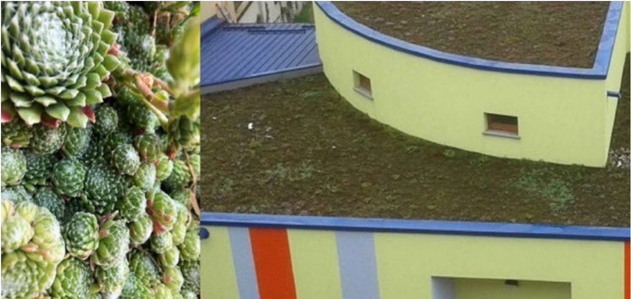
Figure 14: Extensive green roof - sedum, sempervivum - Paguro Children playhouse, Torino (Photo: A. Aires).
