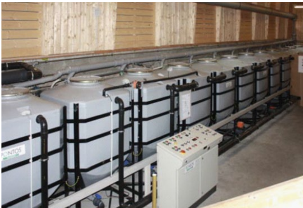
Figure 12: A multi-stage moving bed biofilm reactor (MBBR) for greywater recycling in a residential building (Photo: E. Nolde).
