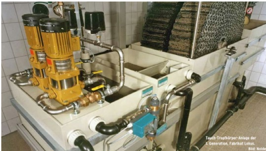
Figure 11: Rotating biological contactors (RBC) in a multi-storey building. First-generation system for greywater recycling from 1995 (Photo: E. Nolde).
