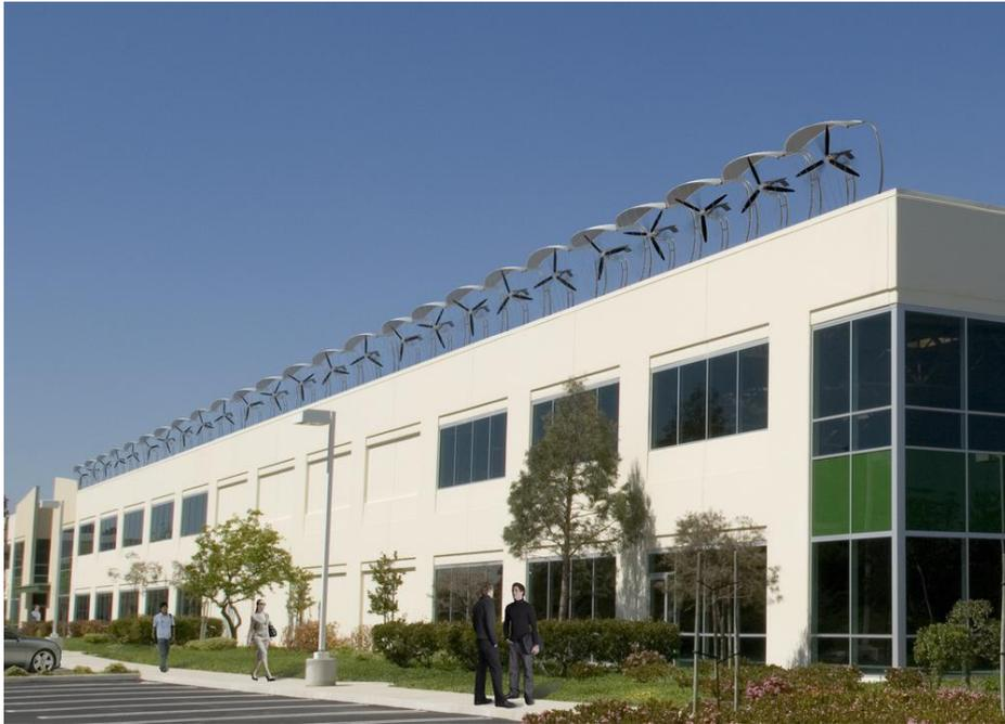
**Picture 8** *Micro windturbines integrated within the urban zone environment*
