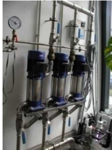
Planted soil filter inside the building
