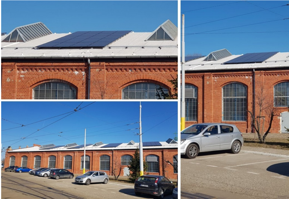
Figure 12: The PV installation on the top of the roof of tram depot of MPK Wrocław (Photo by Marcin Wolek)
