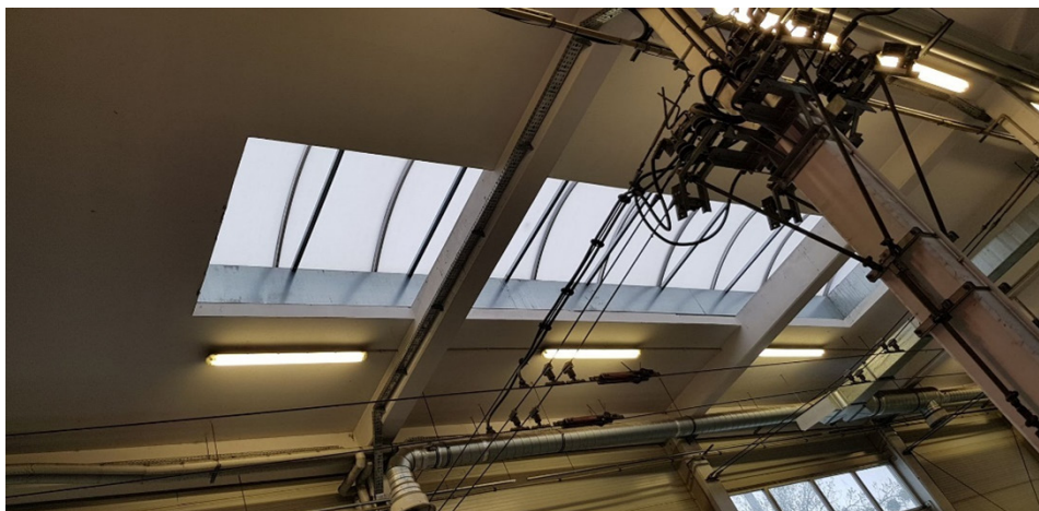
Figure 11: Roof skylights replaced at the depot of PKT Gdynia (Photo by Marcin Wolek)
