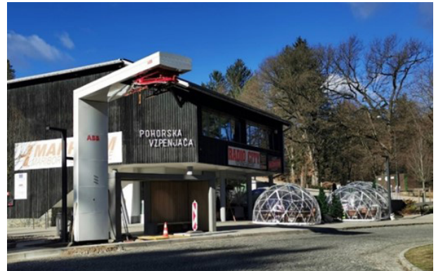
Figure 4: Fast charger for e-buses at the cable car station (Municipality of Maribor)
