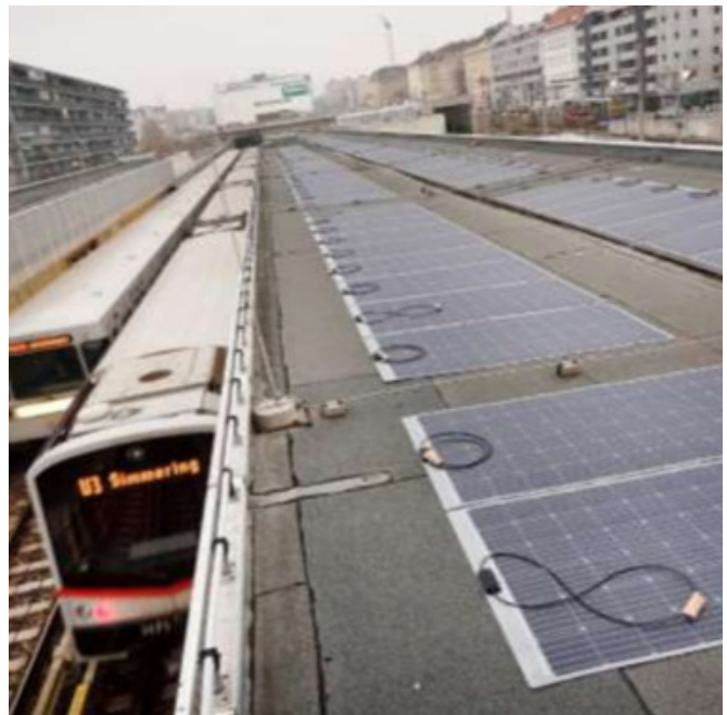
Figure 8: PV-foils on the roof of the metro station (Wiener Linien)
