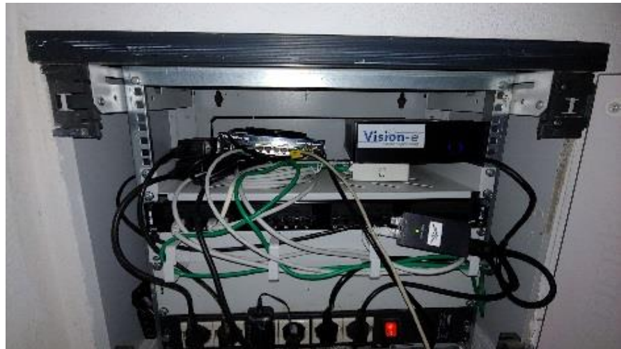
Fig. 6a,b - ENEL concrete pole with the three cameras installed (a) and monitoring equipment in Cà Rossa: the industrial PC is the small box with the label Vision-e, on the top right of fig 6b.
