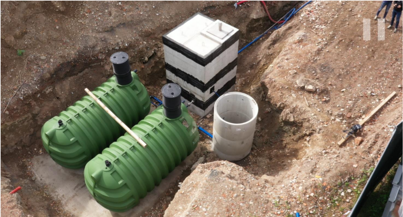
Figure 2: Storage tanks, equipment shaft and pipeline during installation works before backfill
