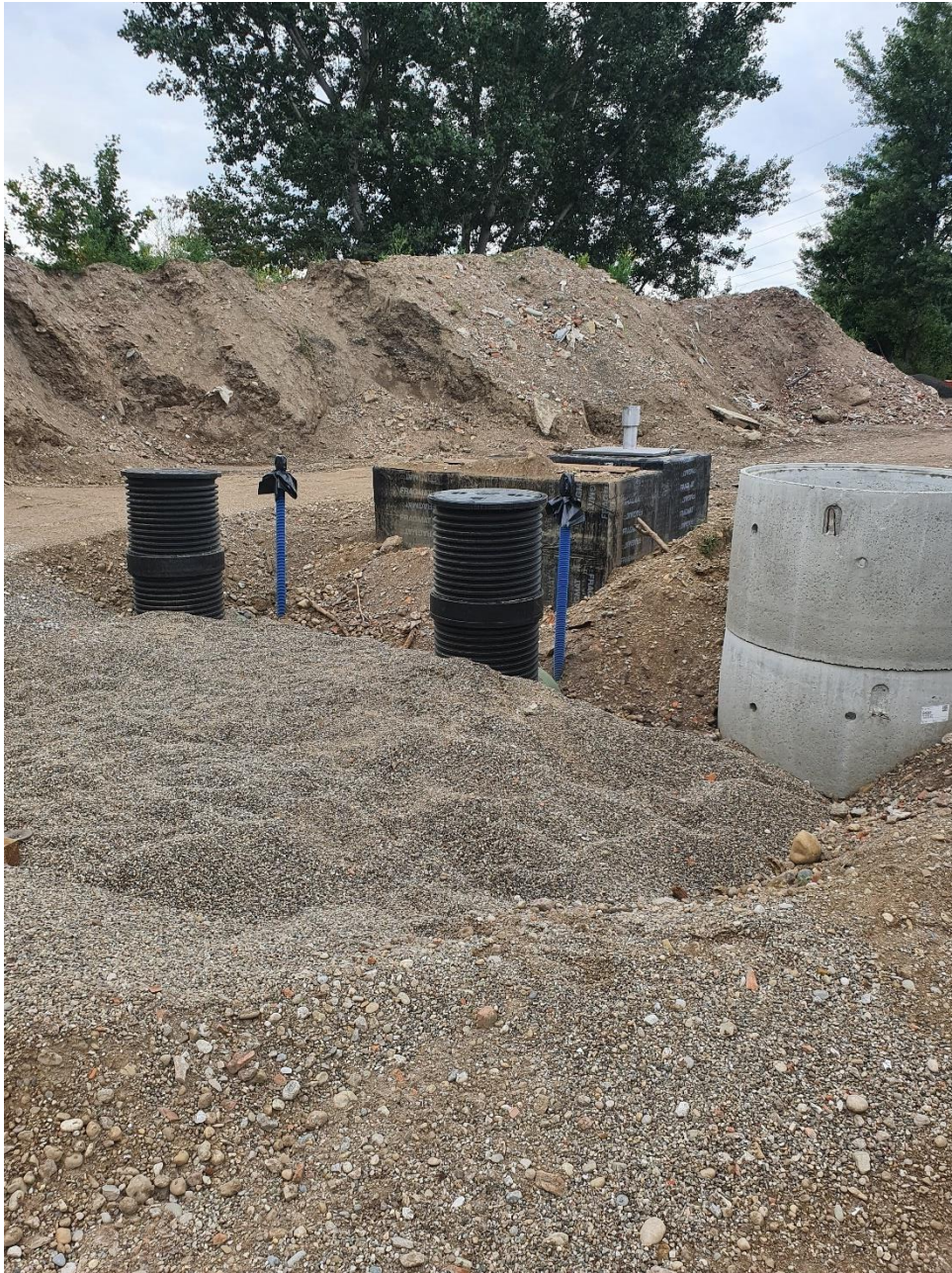
Figure 5: Storage tanks and equipment shaft after most of the land works
