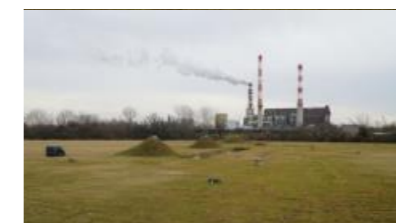
POLAND Tarnów Waterworks
