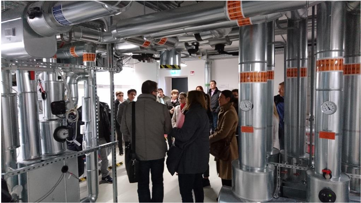
Figure 2: Geothermal heat pumps in the cellar of the Uhlandschul
