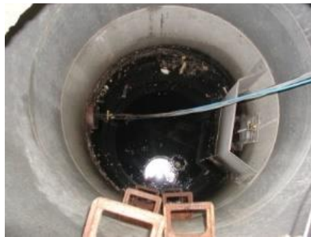
Rainwater sewer with switch diversion
