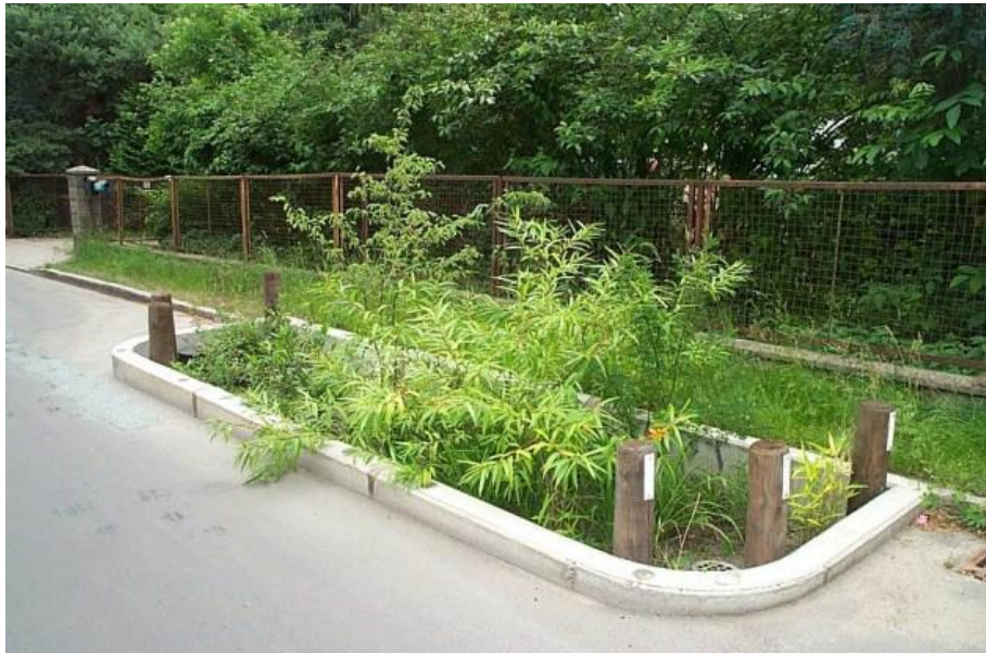
Swale-trench-deep bed system in Birkenstein, Brandenburg (Photo: Sieker)
