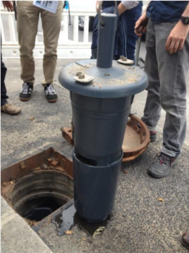
Different systems of decentralised rainwater pre-treatment at Clayallee, Berlin (Photo: KWB, Sieker)
