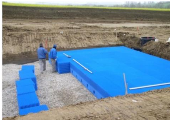
Setup of an infiltration trench with filling material (Photo: Sieker)
