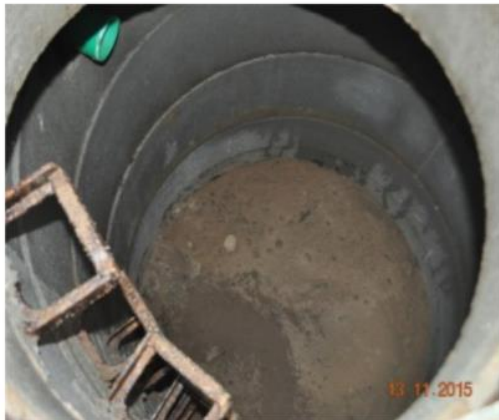
View of the bottom of a soakaway (Photo: Sieker)
