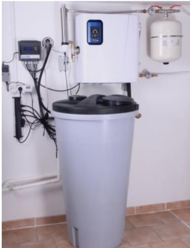
Clear water tank with Rainmaster Favorit SC, AQUALOOP control system and UV disinfection
