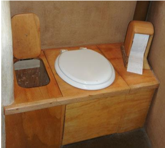
Sawdust composting toilets (waterless)
