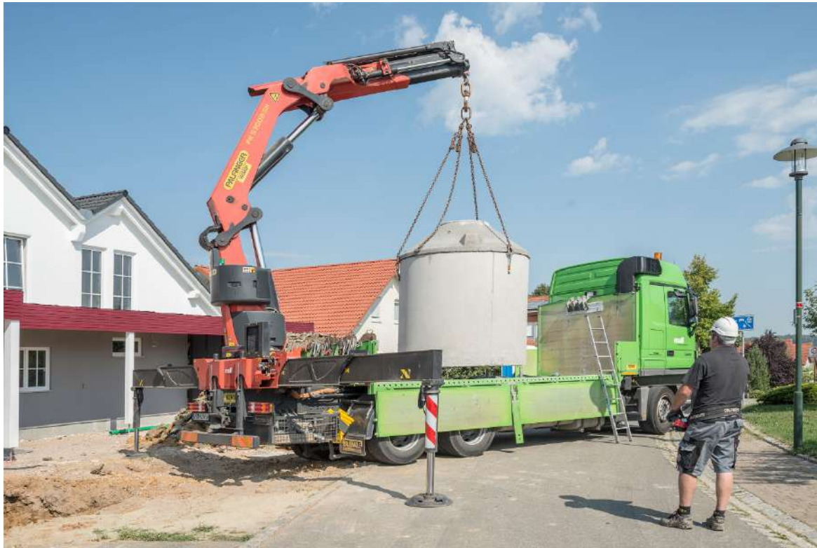
Podzemni spremnik (Mall)
