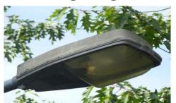
Typical technical luminaire with 50 W HPS lamps
