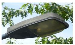
Typical technical luminaire with 70 W HPS lamps
