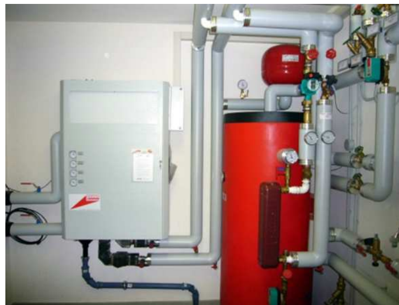
Picture: heat transfer station and hot water storage
