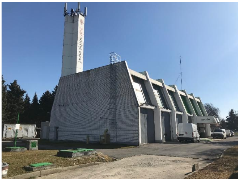
Main boiler room - EO1
