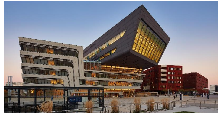
Campus of Vienna University of Economics, 3 MW open loop system for heating and cooling (source: https://www.wien.info/en/sightseeing/architecture-design/wu-campus )
