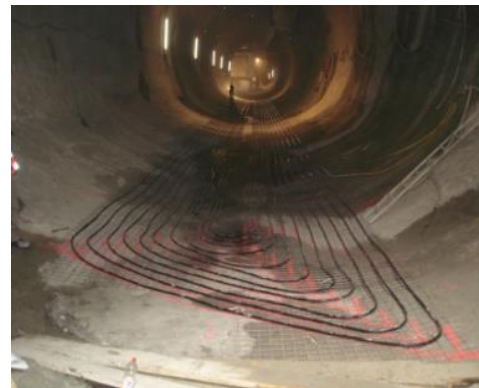
Heat extraction at the underground line U2 in Vienna © R. Markiewicz, 2008
