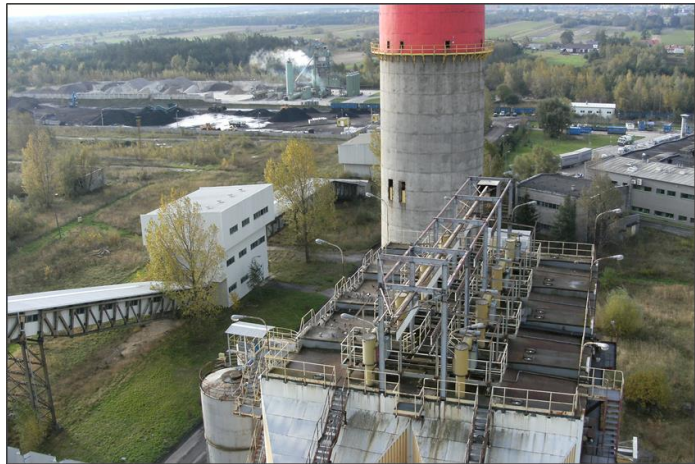
Picture 1 Heating plant in Radom
