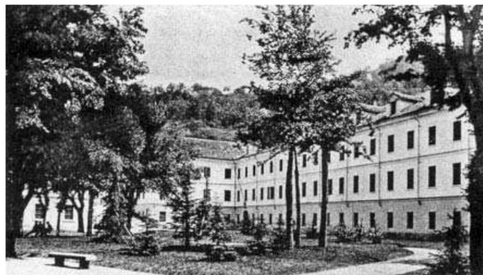
Fig. 2 -The main front of the Military Thermal establishment on the other side of the Bormida, early twentieth century and the Lake of Springs within the Former Military Baths
