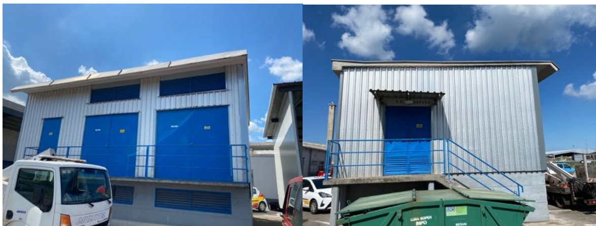
Figure: Existing transformer station
