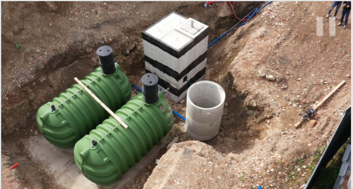
Figure 1: Underground storage tanks and equipment shaft during construction
