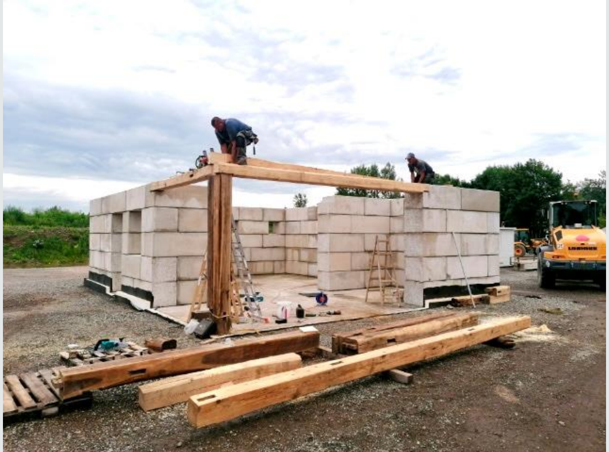
Figure 3: Concrete blocks made from SRM (secondary raw materials) including recycled water provided through pilot investment
