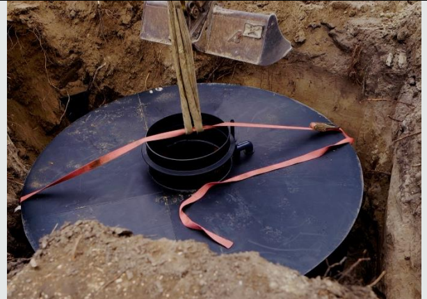
Water tank embedding
