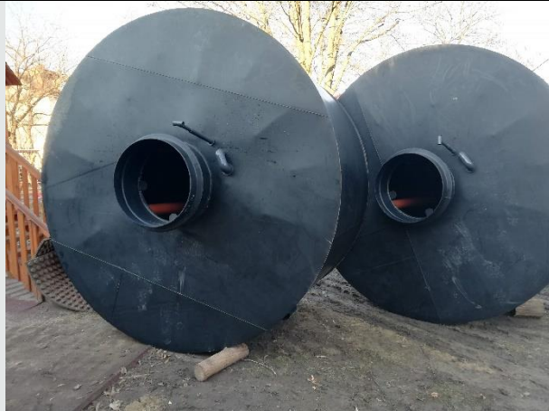
Water tanks (2x7 m3)
