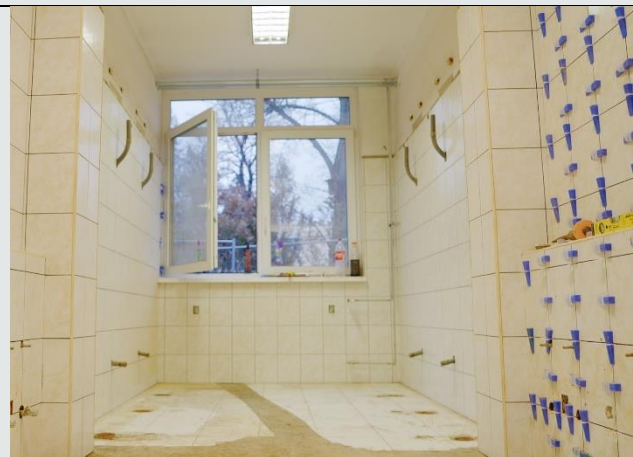
Indoor construction works
