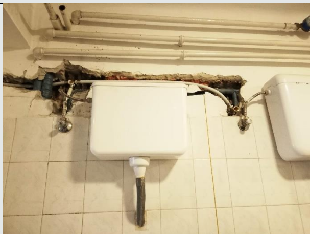
Indoor construction works
