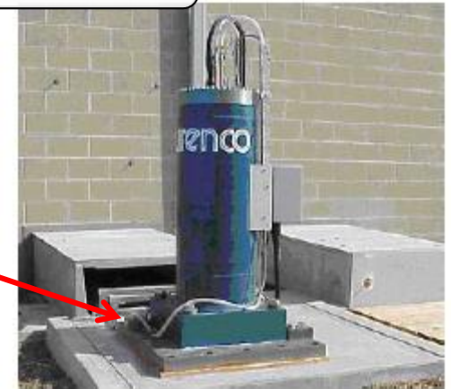
High speed vertical shaft flywheel. Source: Satcom power system
