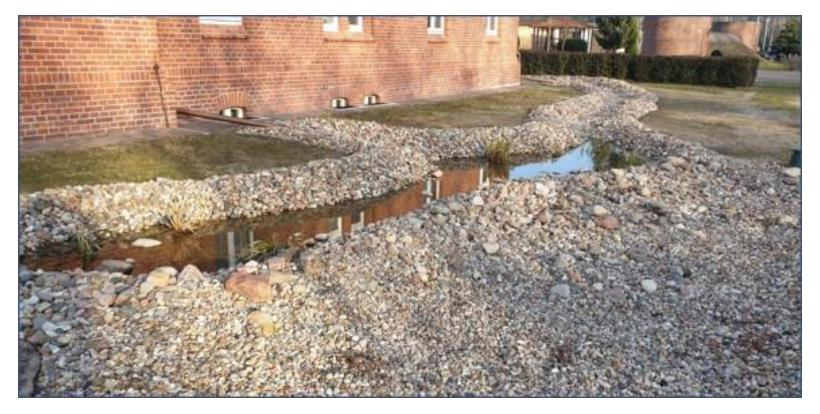
a two-zone rain garden in the ground with a total area of 20.5 m<sup>2</sup> and a capacity of 6.2 m<sup>3</sup>
