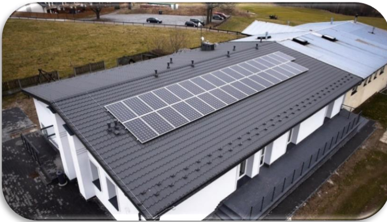
Installation of renewable energy sources systems in public utility buildings and private households (best practice) in Niepołomice, Poland – © Łukasz
