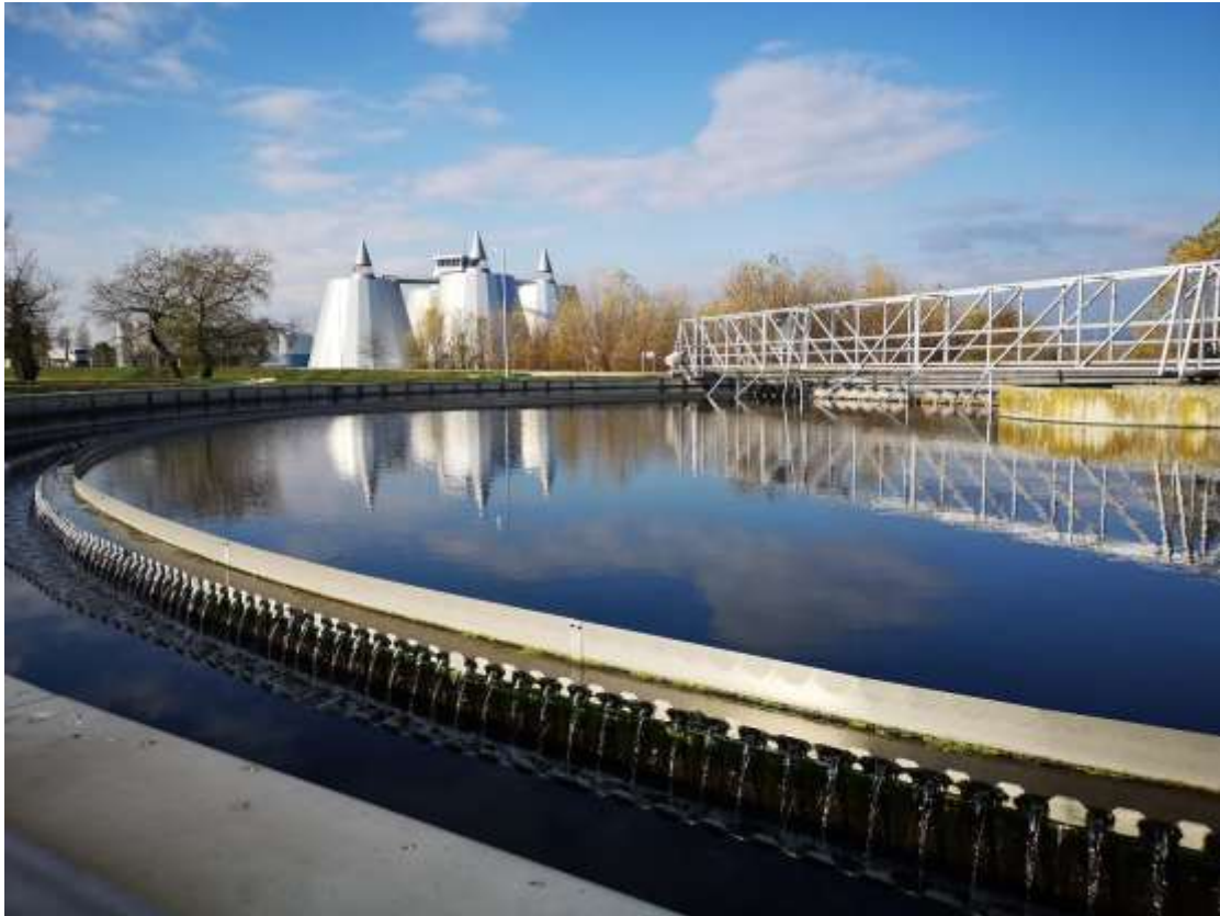
Picture 3: Wastewater treatment plant in Zagreb
