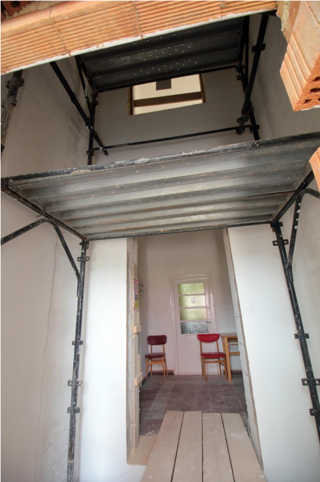
Fig. 6: Works implementation - building the shaft for the elevator
