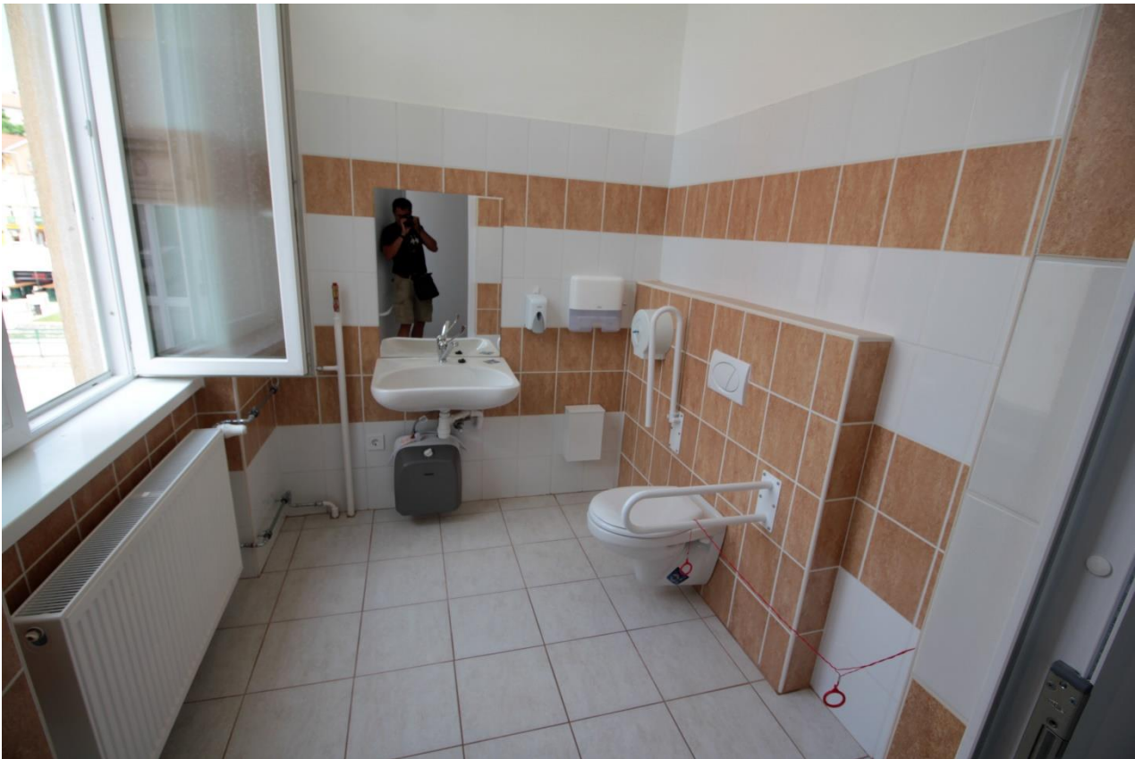
Fig. 5: Second floor barrier-free bathroom
