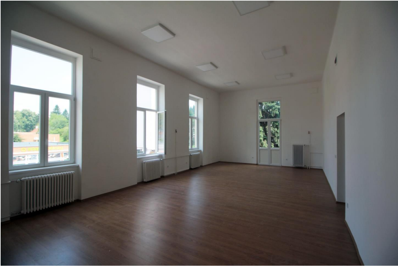
Fig. 5: Works implementation execution of the exhibition hall - the building activity has been finished
