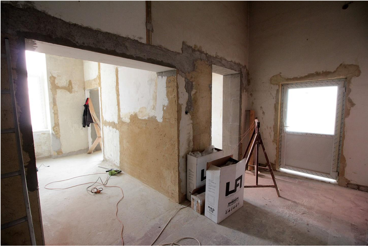
Fig. 2: Second floor creation of Exhibition hall uniting two rooms for the hall
