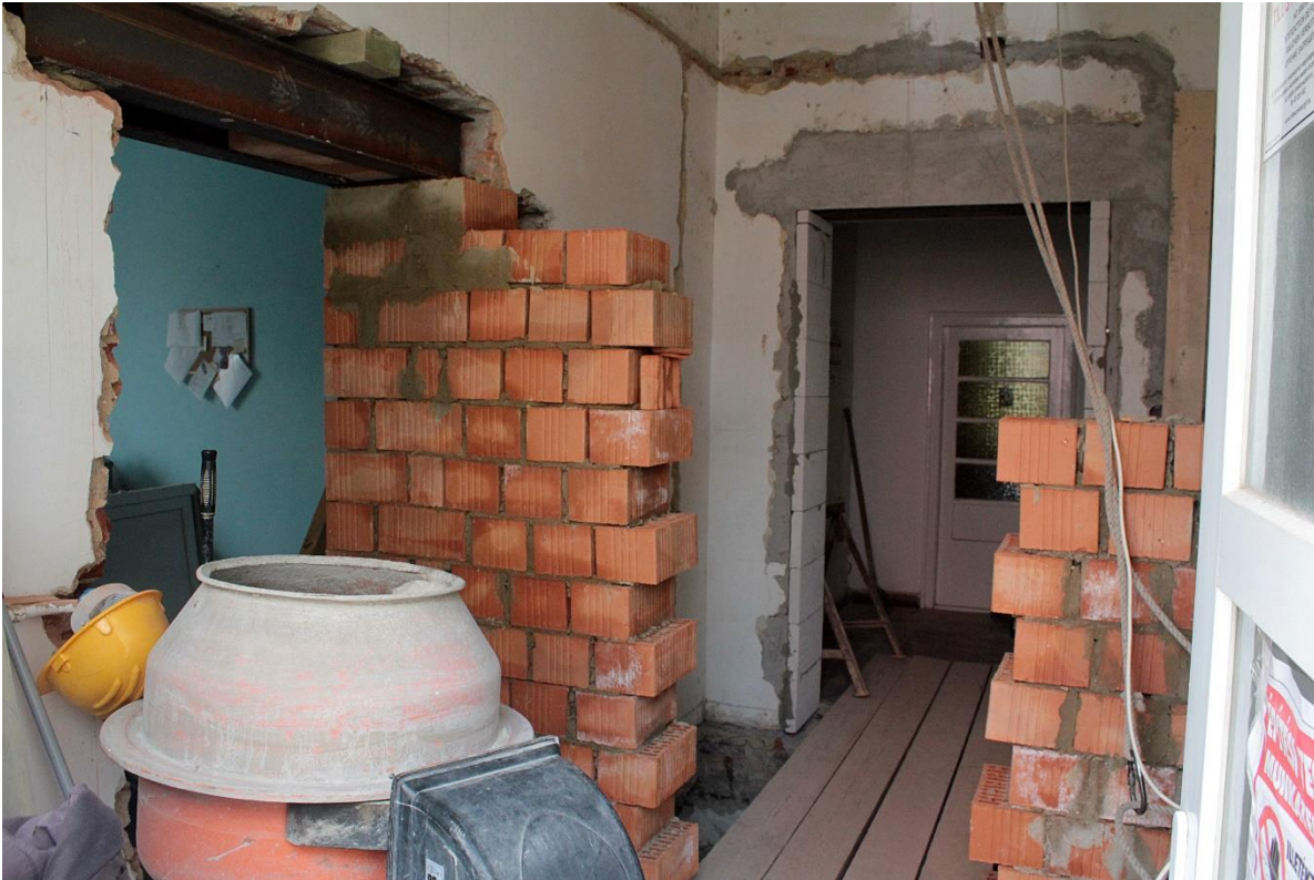
Fig. 1: The elevator's shaft
