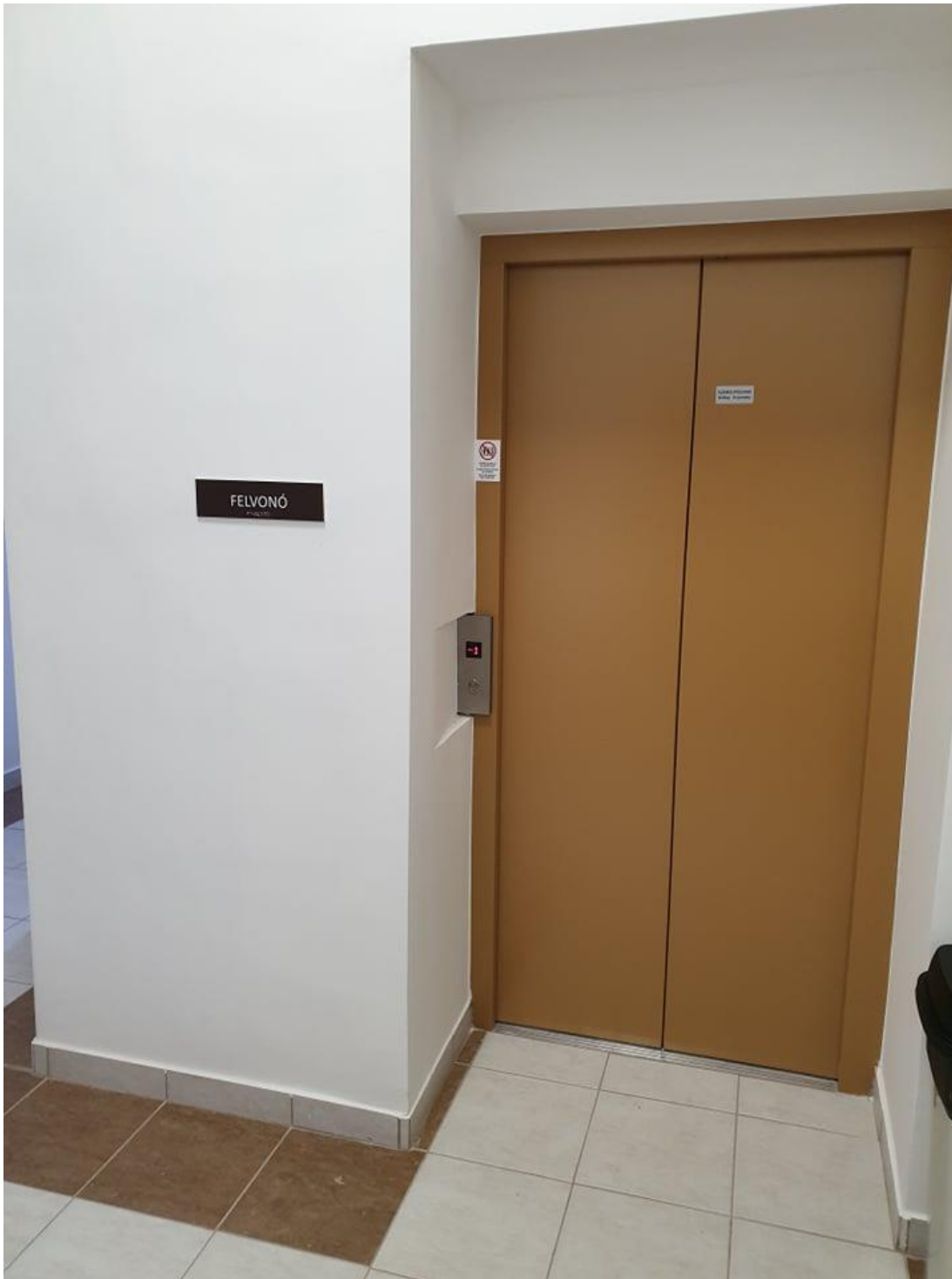
Fig. 5: The barrier-free elevator is ready for usage. The pictograms are also placed on the wall
