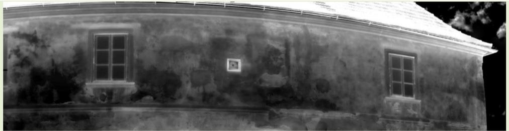
The older interventions in the masonry (walled up windows and arches) are clearly visible
