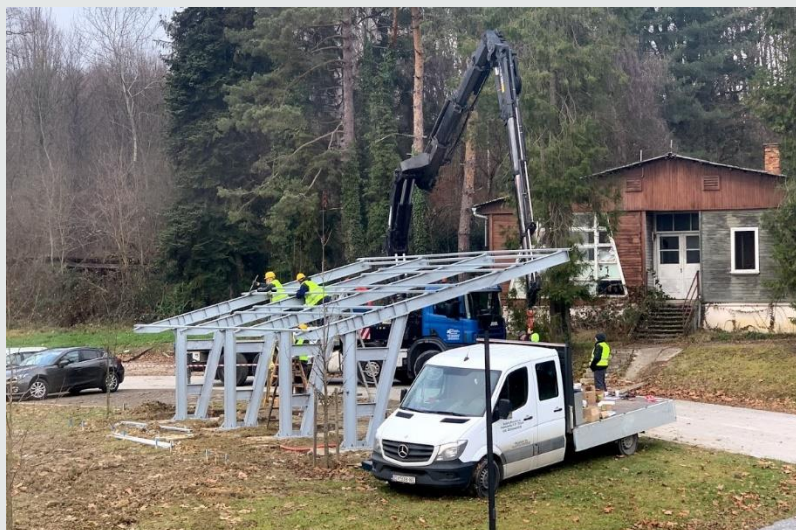
Figure 2: Canopy construction Source: REGEA 2021.
