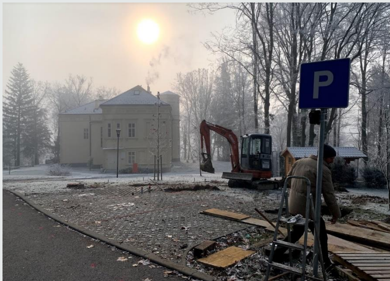
Figure 1: Preparatory works Source: REGEA 2020
