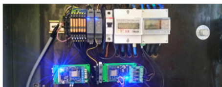
Smart metering system in kindergarten Optica Koprivnica, Koprivnicko - krizevacka County, Croatia
