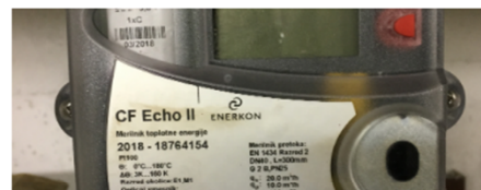
Smart metering system in public building "Music Scholl Fran Korun Koželjski Velenje" Velenje, Savinjsko-Saleška region, Slovenia
