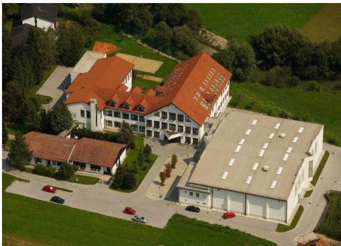
Figure 2 - pilot building in Municipality of Nazarje (SI)
