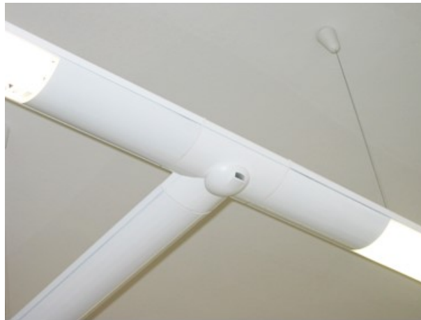
Figure 6.7: Modern fluorescent lighting with DALI control
