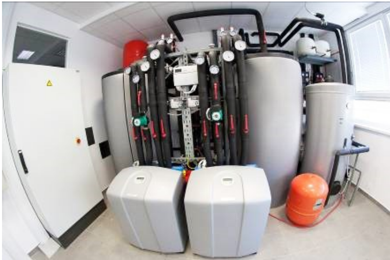
Figure 6.6: The combination of hot and cold water storage tank, boiler and reversible heat pump in thermal substation
