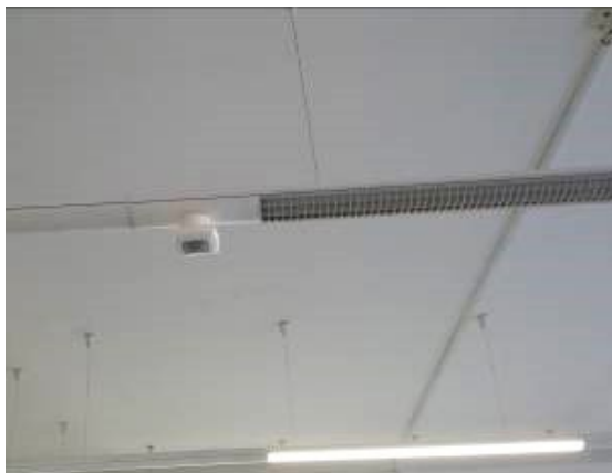
Figure 6.8: Occupancy and lighting sensor; lighting control cabinet with 4 scenes
