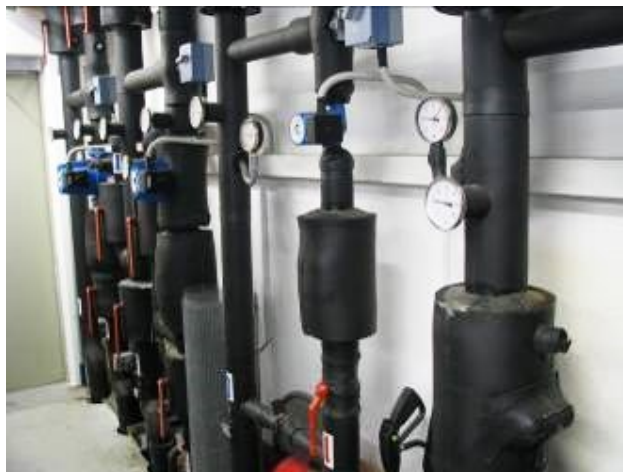
Figure 6.5: Modern distributor of hot water
