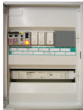
Figure 6.8: Occupancy and lighting sensor; lighting control cabinet with 4 scenes
